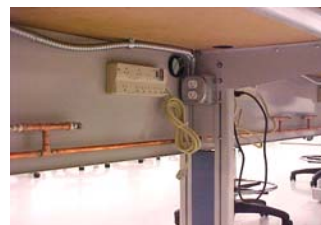
Utility run under worksurface, thru columns
