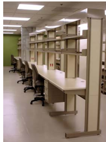
Overhead utility chase on wide column bench row
