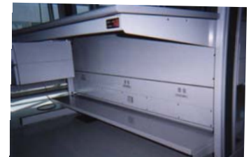
Enclosed utility chase under worksurface
